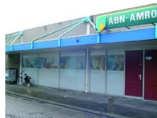
Figure 5.81 Exterior after second upgrade
