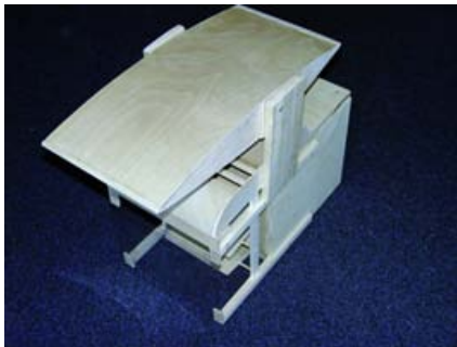
Figure 4.16 Model of double skin facade of wood
