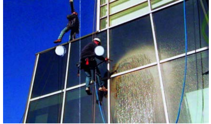
Figure 5.59 Testing of air and water tightness on location
