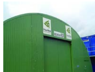
Figure 6.20 Shed with mockup of laboratory room
