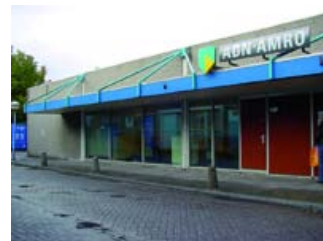
Figure 5.77 Exterior after first upgrade
